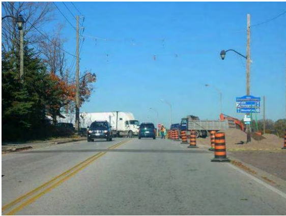
Photo 8 - 25: Guelph Line, near construction zone at Highway 401 Interchange
