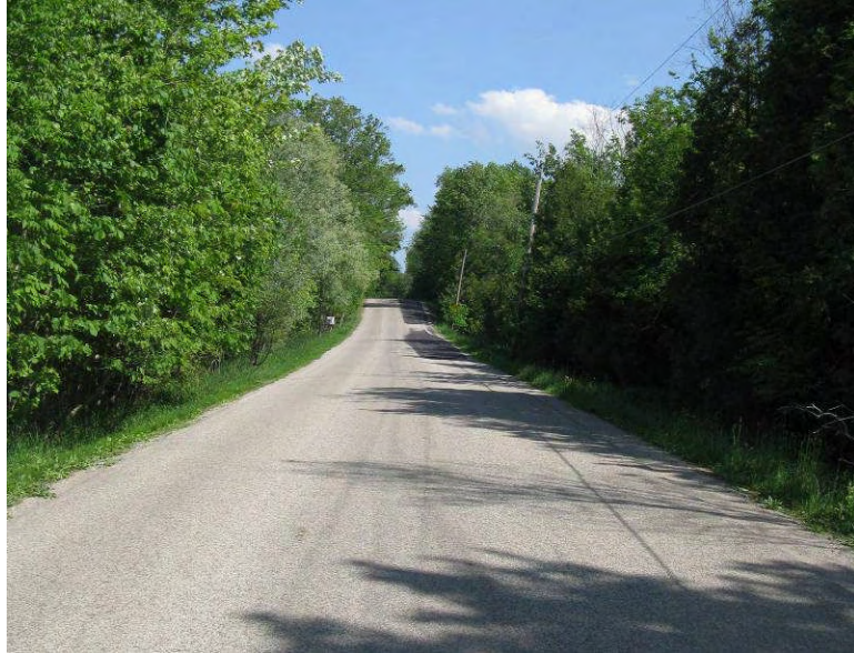
Photo 8-59: Horizontal Alignment along Milborough Line between Concession 11E and Campbellville Road
